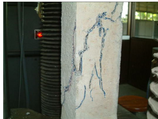
Figure 2. Cracks and spalling of concrete covering on column CB3.2
