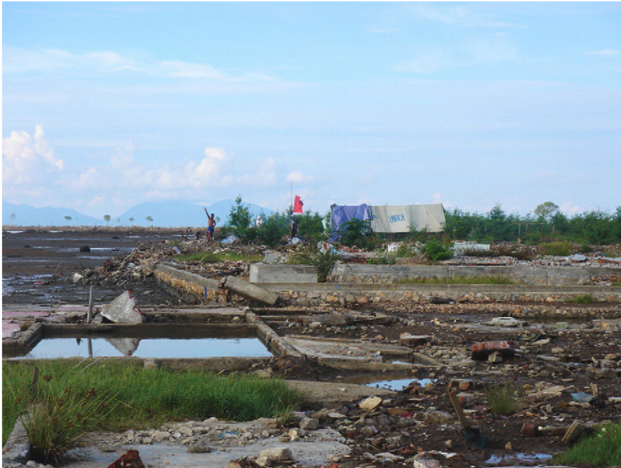
Fig. 14. Severely damaged coastal area and tidal flat in Banda Aceh. Photo was taken at low tide on Dec.1, 2005.
