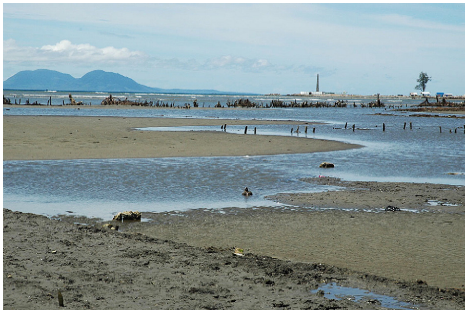
Fig. 13. Severely damaged shrimp ponds in the western part of the Banda Aceh coastal lowland. (Dec.1, 2005).
