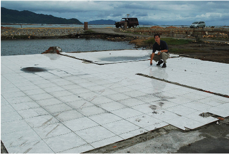
Fig. 6. Scratches on a floor near the coast of the Banda Aceh coastal plain.
