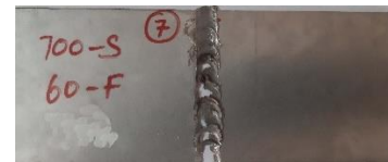
b) Defective welded joints
