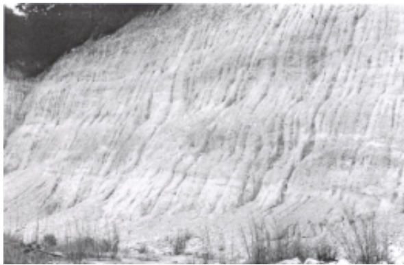
Figure 10. Terrace gravel with erosion along road from Hat Yai to Na Mom.
