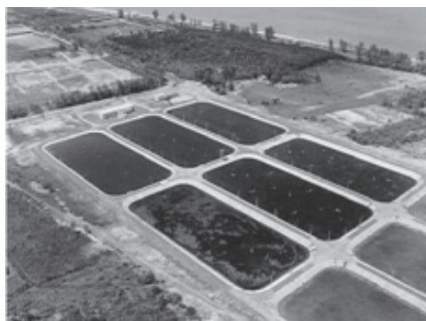
Figure 2. Songkhla central wastewater treatment plant
