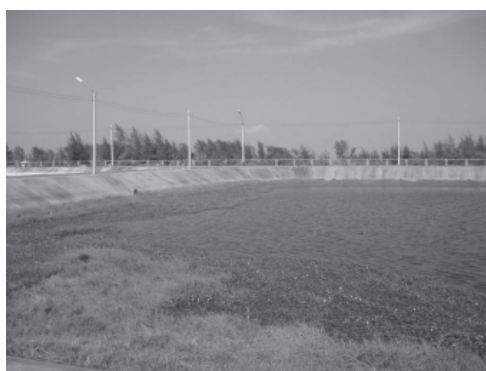
Figure 3. Unwanted plants in the final polishing pond, non-operating
