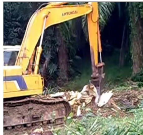
Figure 1. Dead palm tree was ground by backhoe
