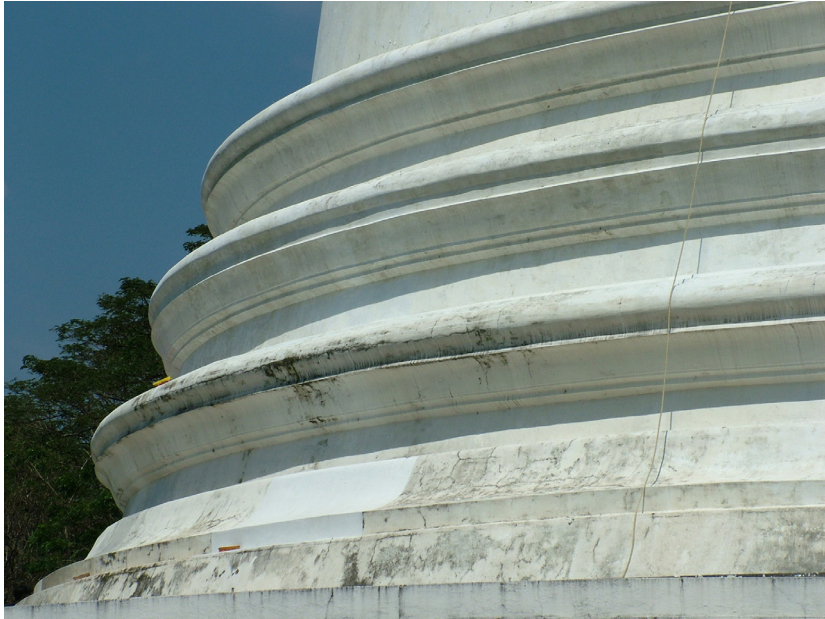
Fig.3 Triple torus moldings of Mahiyangana Stupa, the typical character of Post-Polonaruwa period
