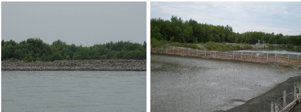
Figure 7 Heightening of Dikes (left) and a Concrete-pole Breakwater (right)
